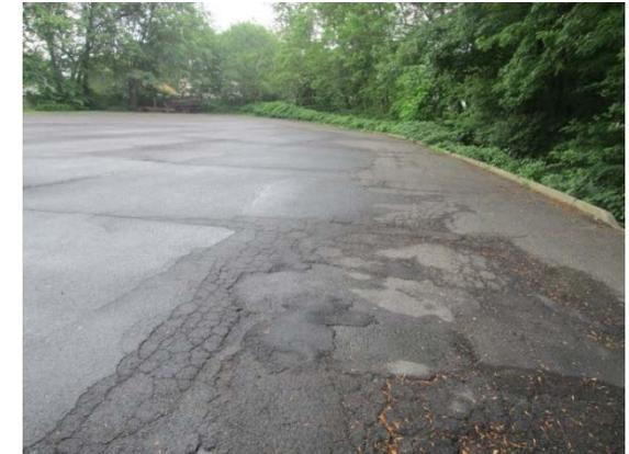
Roof runoff flows into a catch basin at the street and into an adjacent creek. The paved area can be treated with strips of pervious pavement to capture this runoff. Some downspouts can also be routed into a cistern to harvest stormwater and wash the fire trucks. A preliminary soil assessment for this site suggests that soils have suitable drainage characteristics for green infrastructure.
