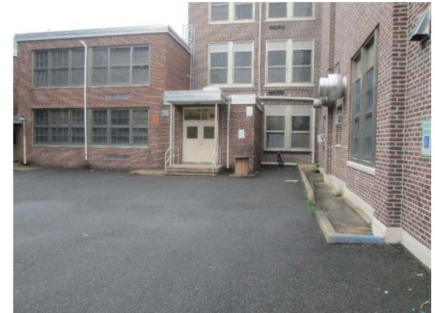
Disconnected downspouts primarily flow directly into street-side storm drains. Porous pavement can be used to capture this runoff. Connected downspouts at the front of the high school can be disconnected into a rain garden. A preliminary soil assessment for this site suggests that soils have suitable drainage characteristics for green infrastructure.
