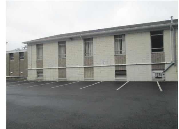
With the exception of the entrance overhang, downspouts currently connect roof runoff directly into the underground sewer system. Downspouts adjacent to the sidewalk can be disconnected into planter boxes, while downspouts by the parking lot can be disconnected into pervious pavement. A preliminary soil assessment for this site suggests that soils have suitable drainage characteristics for green infrastructure.
