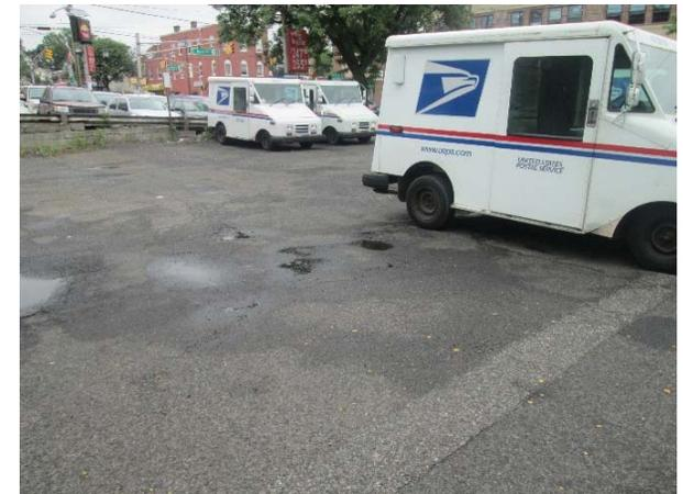
The mail truck parking area has some pooling and erosion concerns and runoff currently flows into the road. Pervious pavement can be used to capture and infiltrate this runoff. The building has internal drainage. A preliminary soil assessment for this site suggests that soils have suitable drainage characteristics for green infrastructure.
